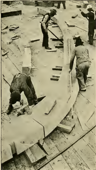
FIG. 51—ASSEMBLING FRAME PUTTOCKS ON FRAMING STAGE
