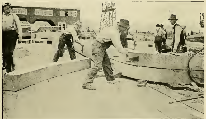
FIG. 52—RESAWING FRAME JOINTS TO A PROPER FIT
