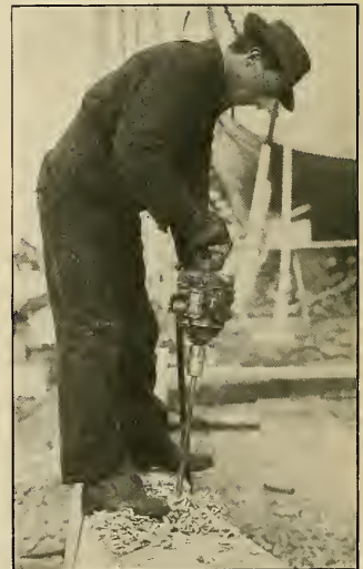
FIG. 11—BORING HOLES WITH AN AIR DRILL
