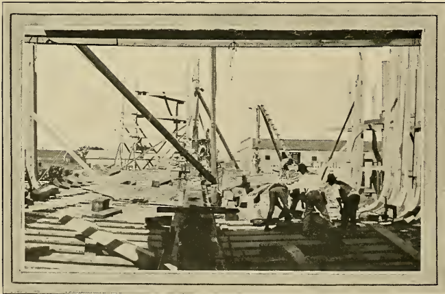
FIG. 98—ARRANGEMENT OF FLOORS, KEELSON AND STEM OF A VESSEL UNDER CONSTRUCTION AT A GULF SHIPYARD
