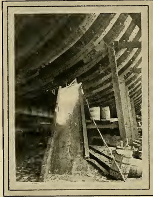
FIG. 131—TIMBER CHUTE FOR HAULING CEILING STRAKES AND KEELSONS INSIDE THE SHIP
