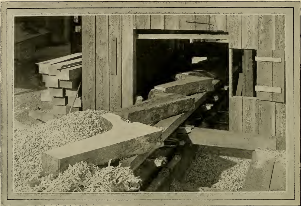
FIG. 174—SURFACING KNEES ON A SPECIAL PLANING MACHINE—KNEES ALSO ARE FAYED ON THIS MACHINE IN LOTS OF 10 OR 12, THE OPERATION REQUIRING ONLY 15 MINUTES
