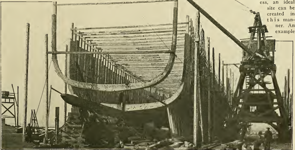
FIG. 16—ELECTRICALLY-DRIVEN, TRAVELING DERRICK SETTING FRAMES IN A WOODEN SHIPYARD
