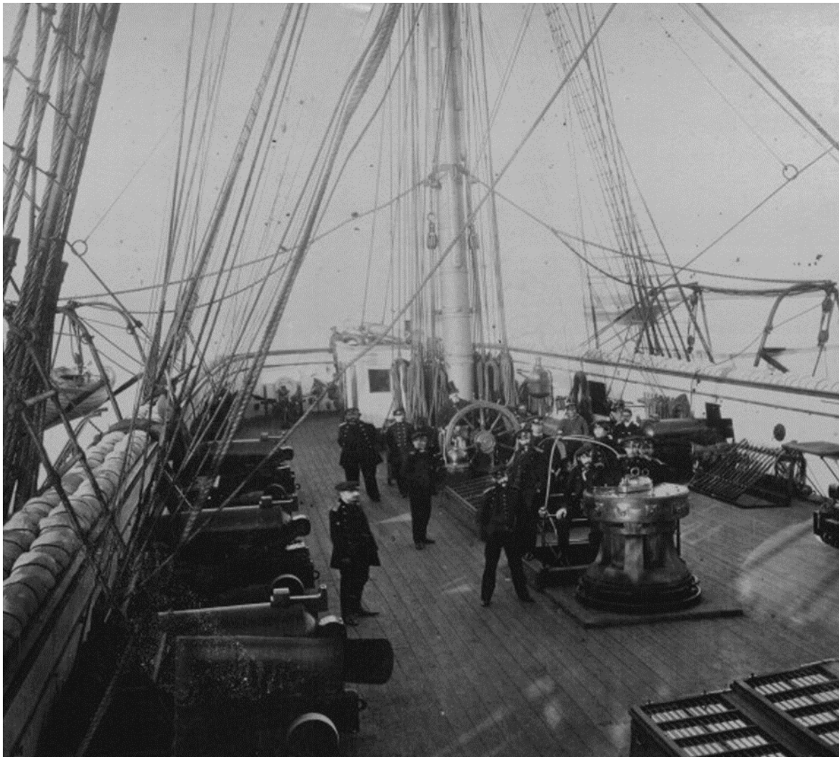
Figure 8 - Running rigging and shrouds "Hawser-Laid", right-handed.
