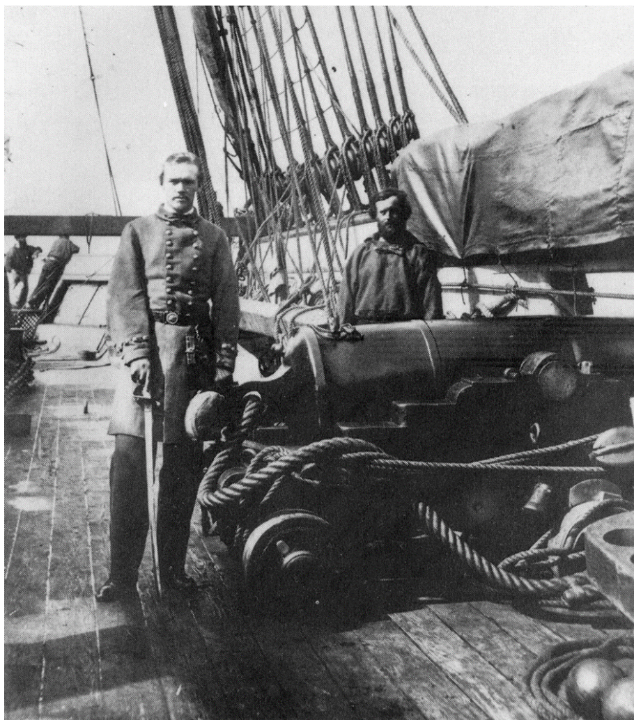
Figure 12 - Running rigging and breeching rope "Hawser-Laid", right-handed.
